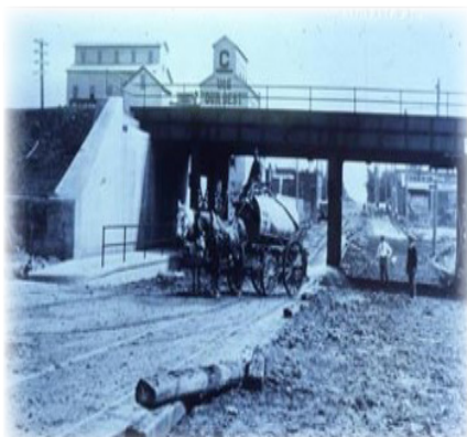
13 Street Underpass, built in 1915 to connect the north and south.
