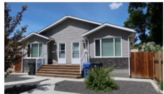
Temporary duplex at 1419 4 Avenue North
