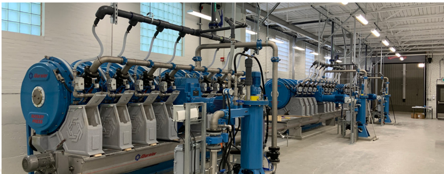
Water Treatment Plant Residual Management Rotary Presses
