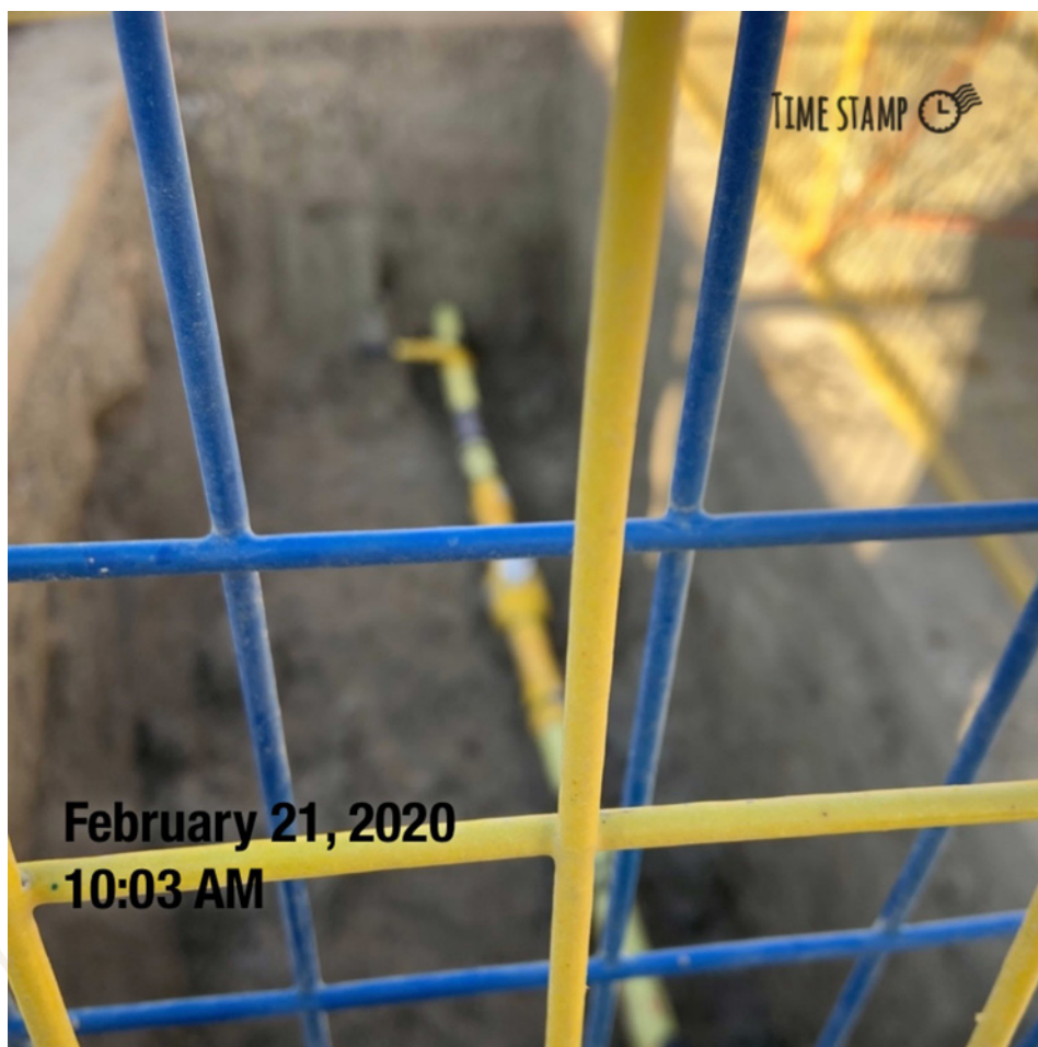
Construction fencing protecting the public and contractor during an Atco Gas shallow utility installation.
