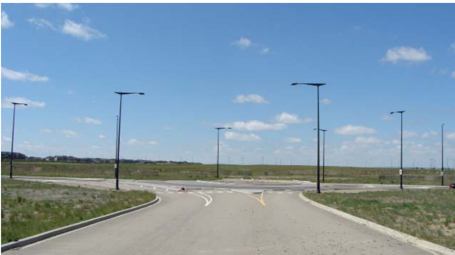
SITE PHOTO LOOKING TOWARDS CENTRAL CROSSINGS
