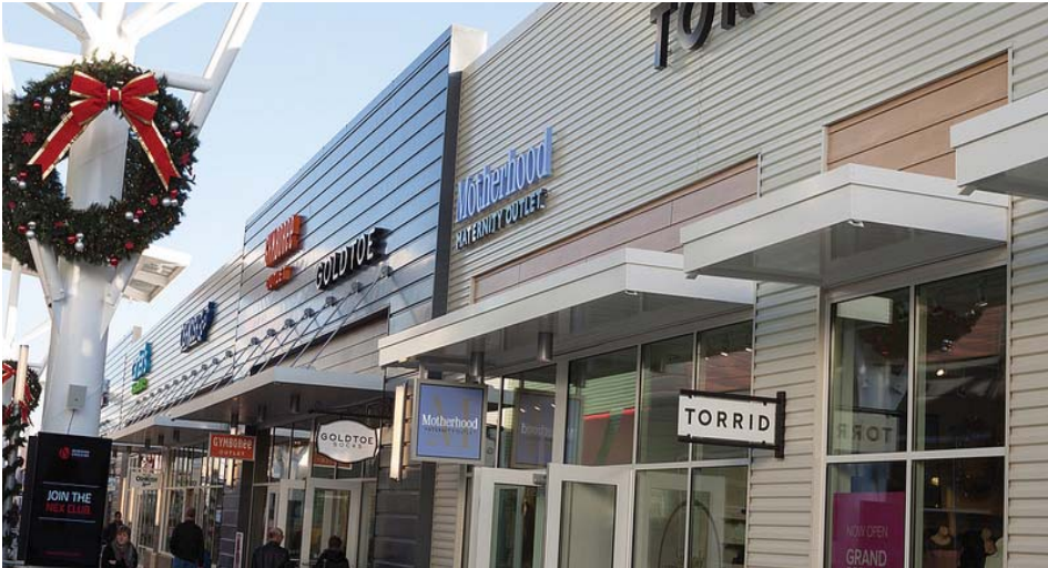
NEBRASKA CROSSING SHOPPING CENTRE, NB (IMAGE B)
