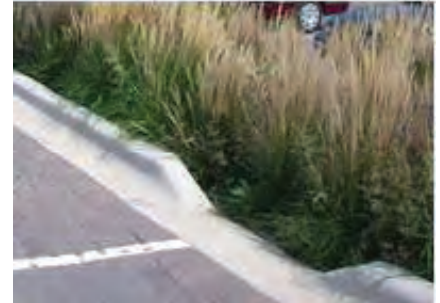
Bio-Infiltration Planting Used to Detain Stormwater Run-Off
