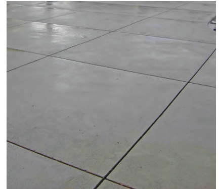
Concrete Sidewalk With Saw Cut Control Joints – Highly Accessible Pedestrian Movement
