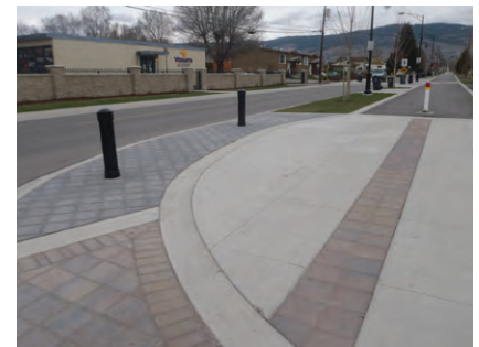
Urban Braille Treatment with High Contrasting Pavers and Tactile Changes at Intersection
