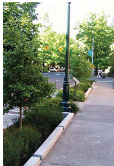
Bio-infiltration Swales and Rain Gardens Help Retain Stormwater and Reduce Infrastructure Costs
