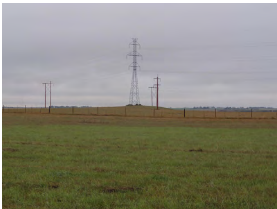
Figure 17: Altalink transmission lines border the cemetery site. LEES+Associates
