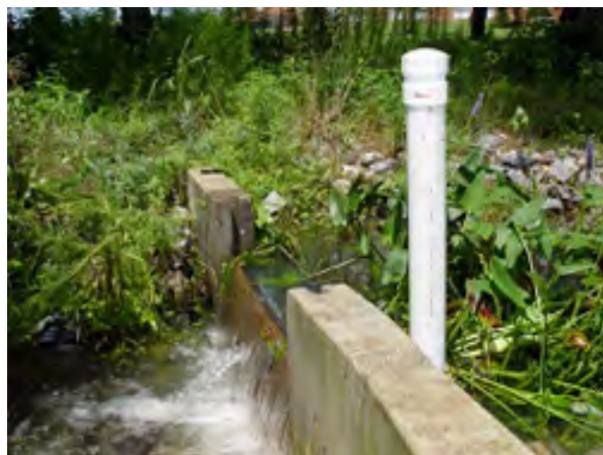
Figure 11. Adjustable outlet structures are modifications of the flashboard riser.
