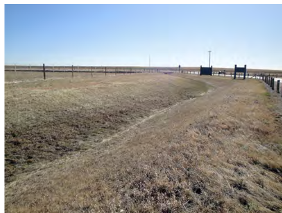
Figure 20: A stormwater berm currently runs along the edge of the site. LEES+Associates
