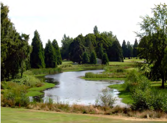
Figure 26: Constructed stormwater detention pond, LEES+Associates
