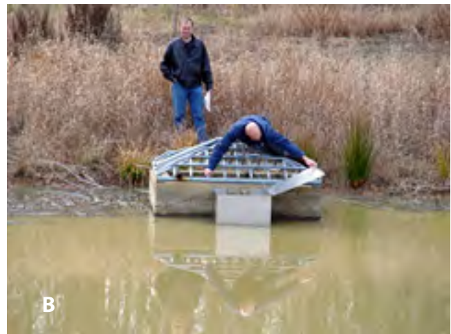
Figure 8. Downturned pipe on an orifice (A) and a trash rack in place around an orifice (B)
