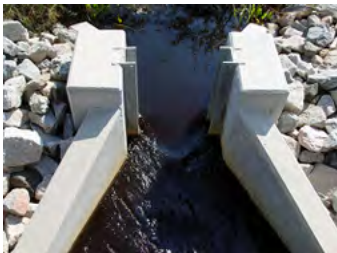
Figure 11. Adjustable outlet structures are modifications of the flashboard riser.
