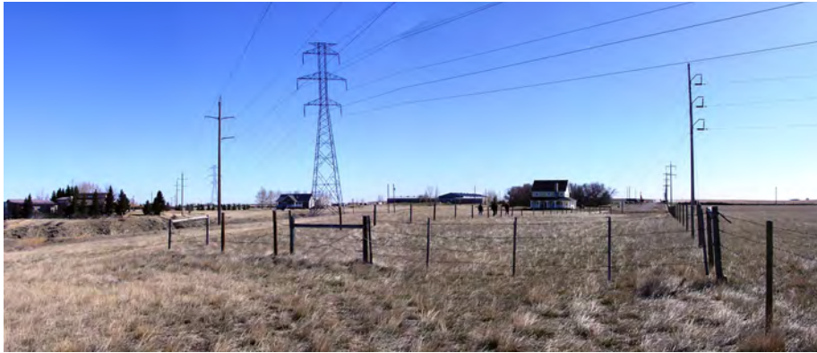
Figure 7: Transmission lines, with the Pavan Family Property in the background, LEES+Associates
