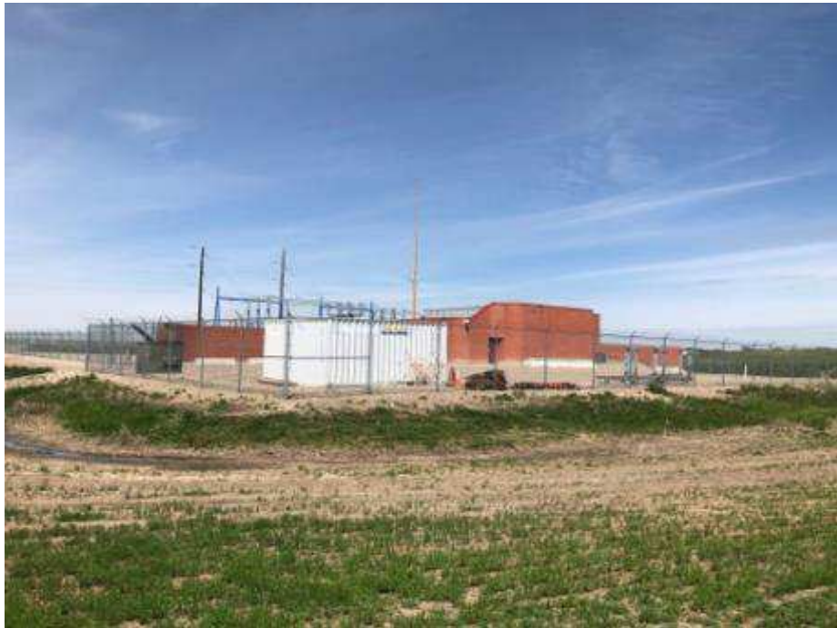
Photograph 8 – Bowron Substation Facing Northwest Note the garbage bin to the left.
