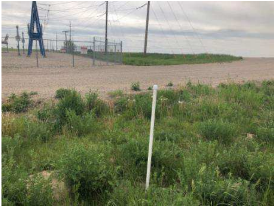
Photograph 11 – Possible Geotech Piezometer on Northern Side of Northern Access Road to Substation
