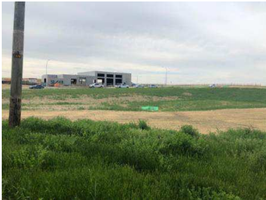
Photograph 28 – New Fire Station Lot Under Construction Facing Southwest
