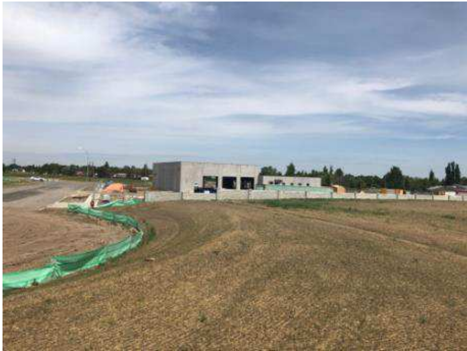
Photograph 33 – Facing North Towards Fire Station
