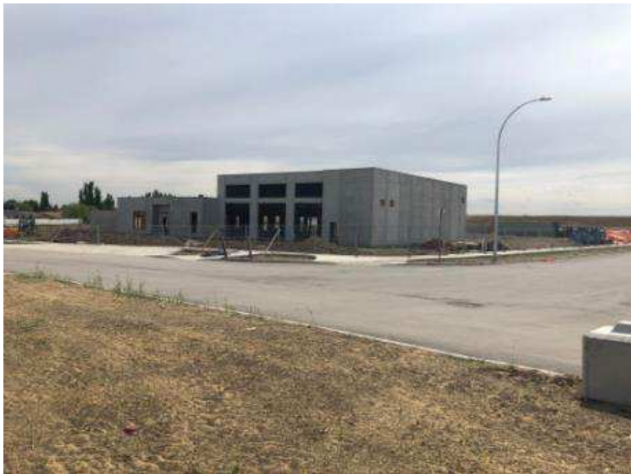
Photograph 32 – Fire Station Building Under Construction Facing Southeast
