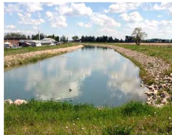
SMRID irrigation canal through SEASP area
