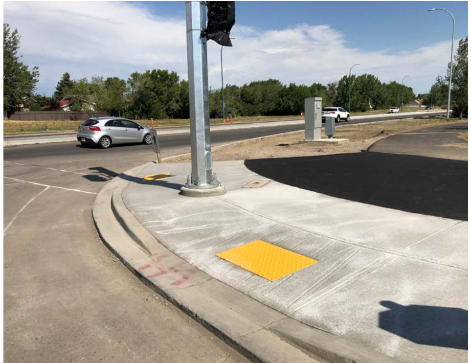
New signal poles and accessibility pedestrian crossing ramps located at University Drive at Grand River Blvd/Rocky Mountain Blvd West.
