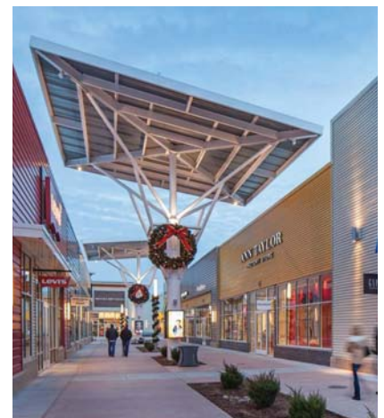
NEBRASKA CROSSING SHOPPING CENTRE, NB (IMAGE G)
