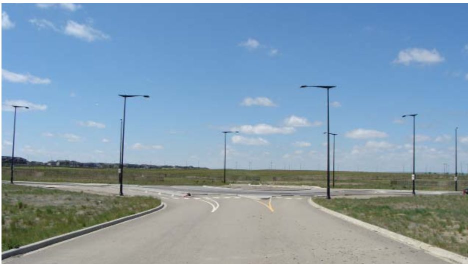
SITE PHOTO LOOKING TOWARDS CENTRAL CROSSINGS
