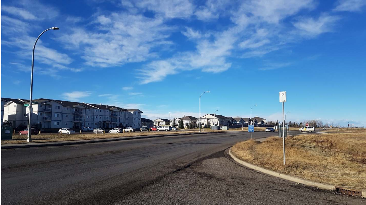
Figure 8-4: RI/RO Access on Walsh Drive – Looking West towards Westside Drive
