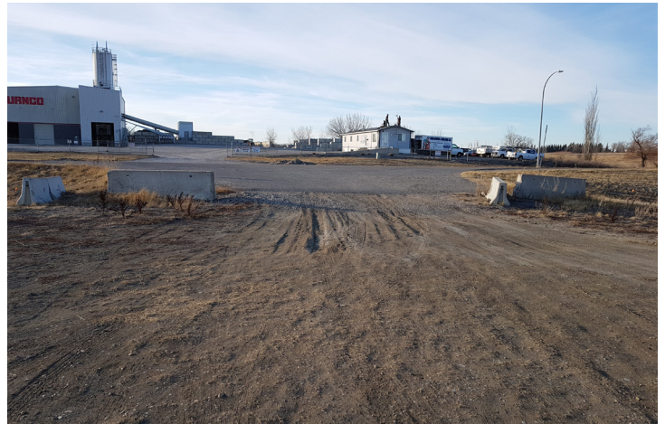
IMAGE 7 - WEST SITE ACCESS - VIEW LOOKING WEST
