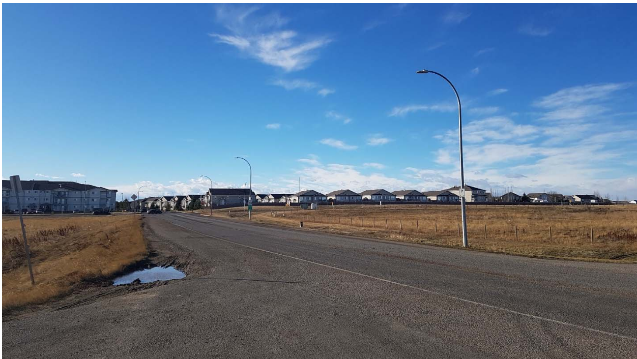
Figure 8-1: Main Access – Looking South towards Walsh Drive
