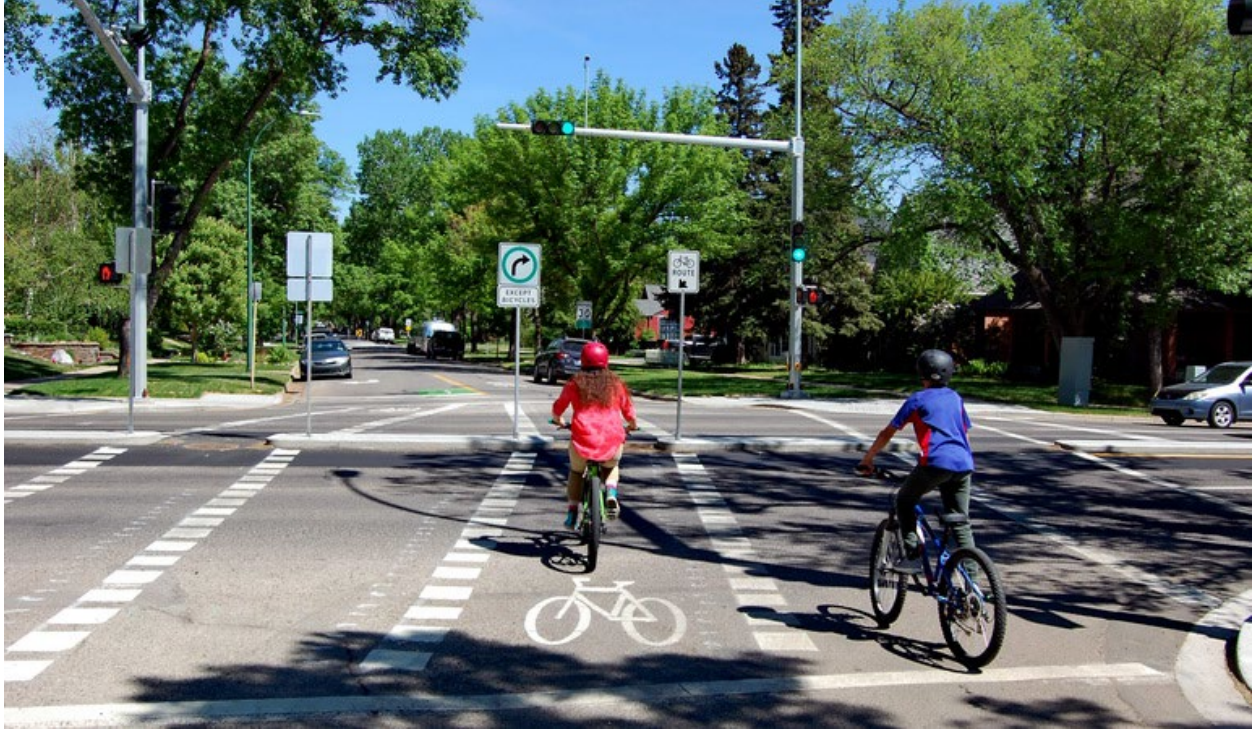
Upgraded intersection at 13 St S and 7 Ave S
