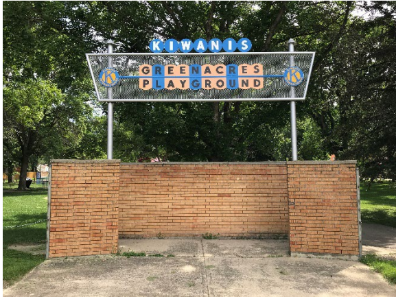
3 Kiwanis Entrance Wall Before
