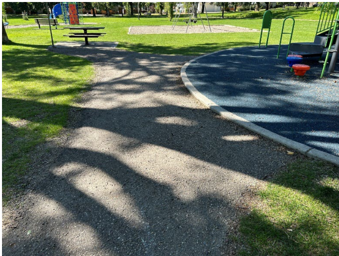
Paving at Kinsmen Park
